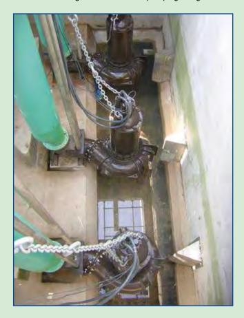
versa immersible pumps are a versatile, innovative development of the established submersible range. Capable of continuous operation in a dry installation, the immersibles may be operated, with equal efficiency, when fully or partially submerged.
