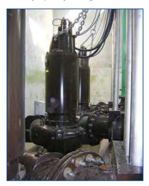
The pumps are particularly suited for dry pit applications where the combination of the Screw Centrifugal Impeller and immersible motor can be considered the state-of-the art technology. Leakage of the pumped product is eliminated by tandem seals running in an oil bath, avoiding a situation commonly experienced with soft-packed glands.
