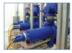
The pumps may be installed vertically or horizontally.
